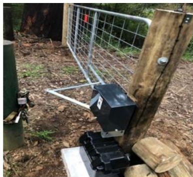
Side Mount Picture: Gates shown here are Opening Out with Motor mounted inside
